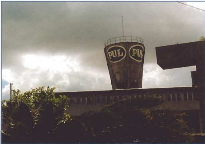
Picture of the Frigorifico PUL (Product of Uruguay) meat processing facility in Melo, Uruguay.
